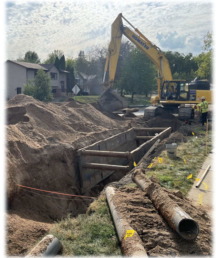
Water main replacement Cope Avenue (2022)
